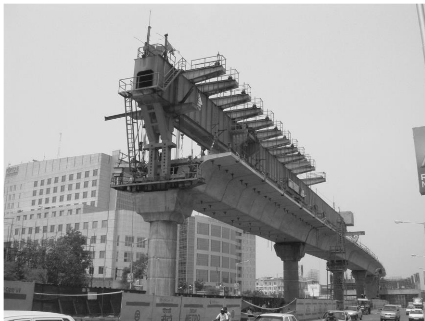
Figure 11 Box Girder Segmental Construction: DMRC Phase 2
