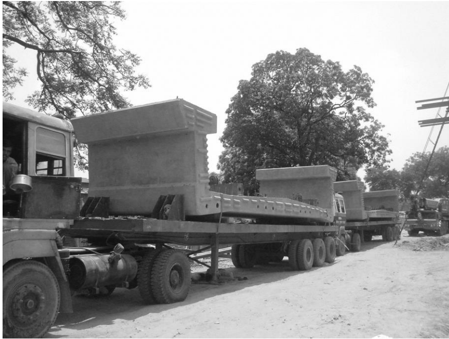
Figure 9 Transportation of segment of 2-track U Girder: Delhi Metro Line
