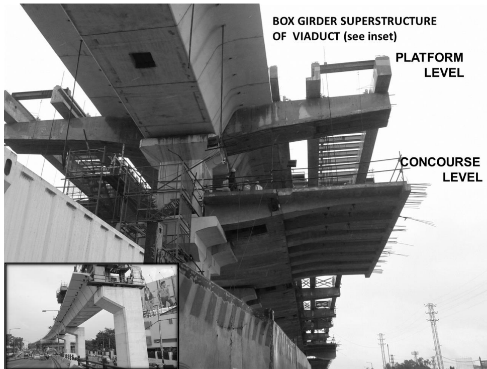
Figure 21 Erection of Precast Elements of Station: Hyderabad Metro
