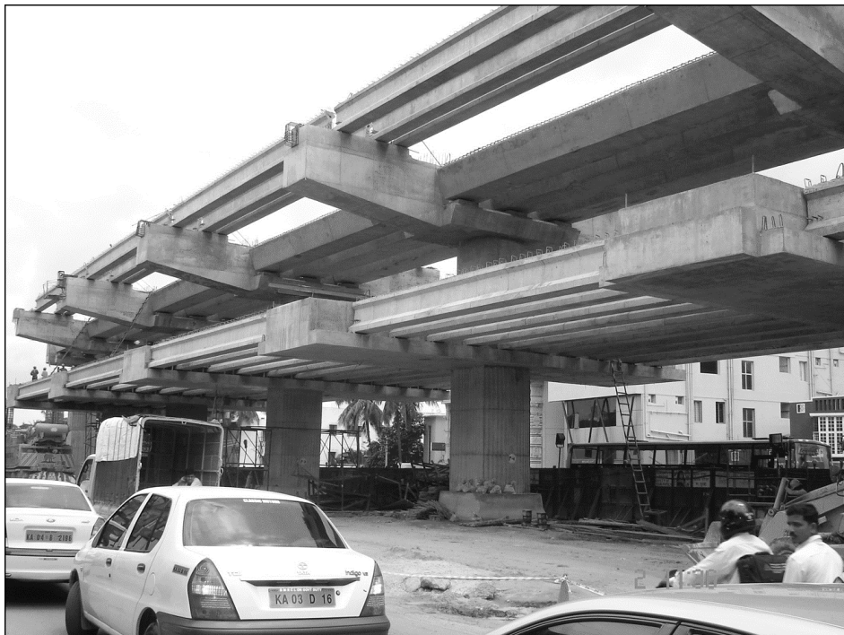
Figure 20 Precast Beams for Platform Level and Concourse Level: Bangalore Metro
