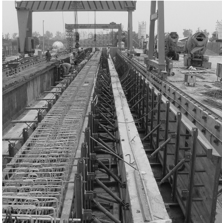
Figure 8 Long Line Casting Beds for Pretensioned Girders: Delhi Metro Phase 1
