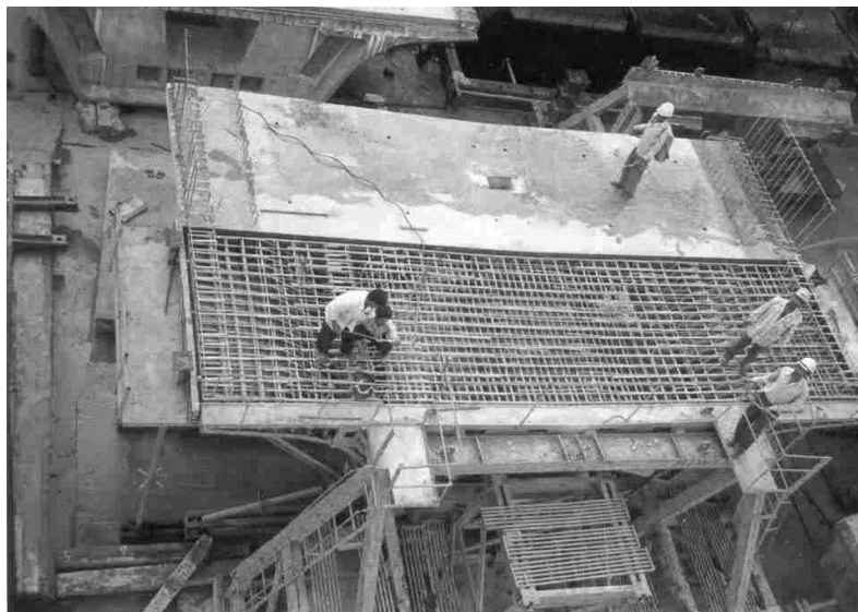
Figure 7 Match Casting Of Segments by Short Bench Method: Delhi Metro Phase 1.
