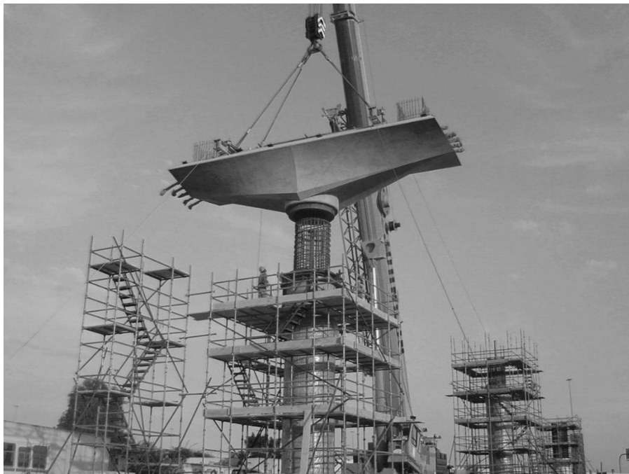
Figure 17 Precast Pier Cap for Twin U-Girder Viaduct: Dubai Metro
