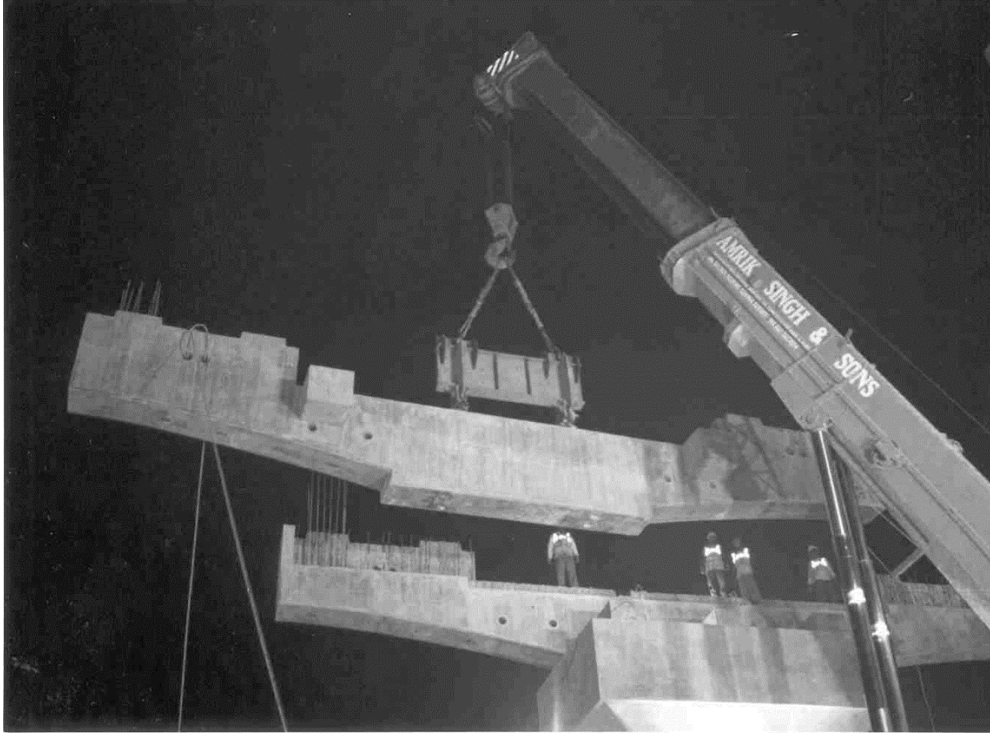
Figure 19 Precast Posttensioned Cross Girder Being Lowered Into Position: DMRC Phase 1
