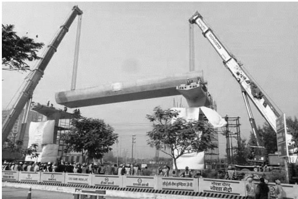
Figure 15 Girder (For 1 Track) Full Span Erection: Noida Metro
