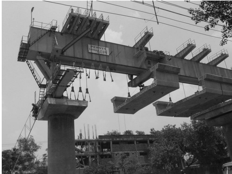
Figure 12 U-Girder (For 2 Tracks) Segmental Construction: DMRC Phase 1
